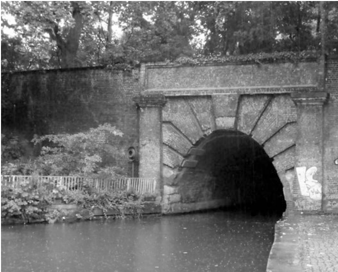
Fig. 1 The Islington canal tunnel, North London. Its effect on 'g', amounting to a few hundredths of a milligal, is just measurable by modern gravity metres on the road above it ( Photograph Anna Milsom )
