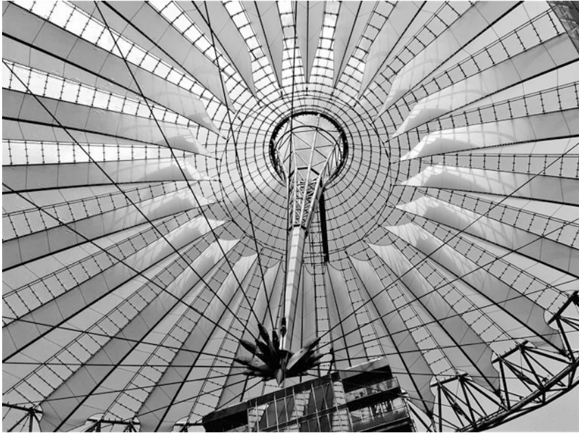
Fig. 1.3 Steel roofing structure of the Sony Center at Potsdamer Platz, Berlin. (Photo: Schlegel, J.)
