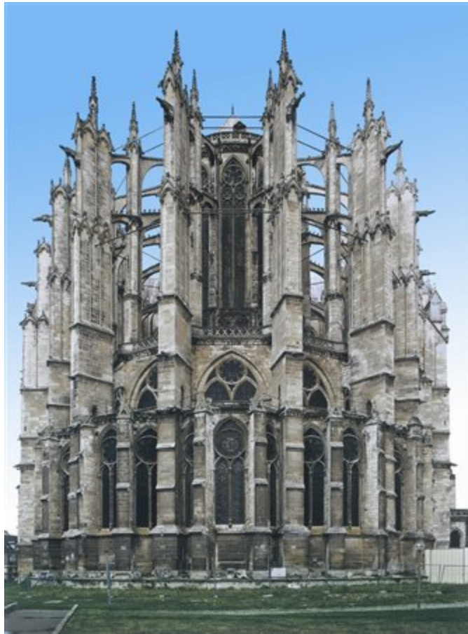
5. Apse, St. Pierre Cathedral, Beauvais (France), begun in 1225 and renovated in 1284 and 1573 after its collapse. In situ.
