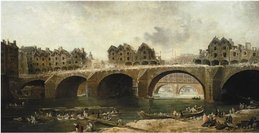
Hubert Robert , Demolition of the Houses on the Pont Notre-Dame in 1786 , 1786.
