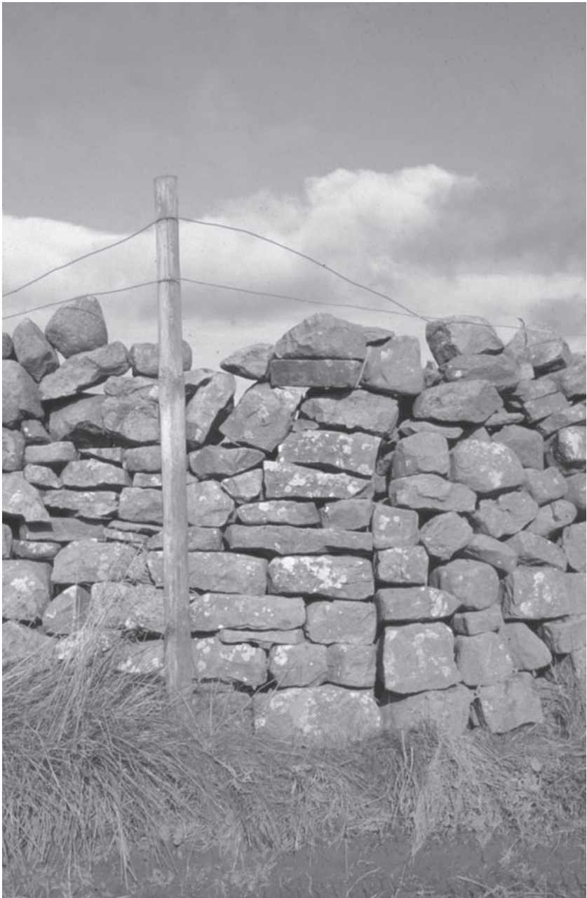
Figure P3 A “butt-joint” in a field wall, near Grinton, Swaledale
