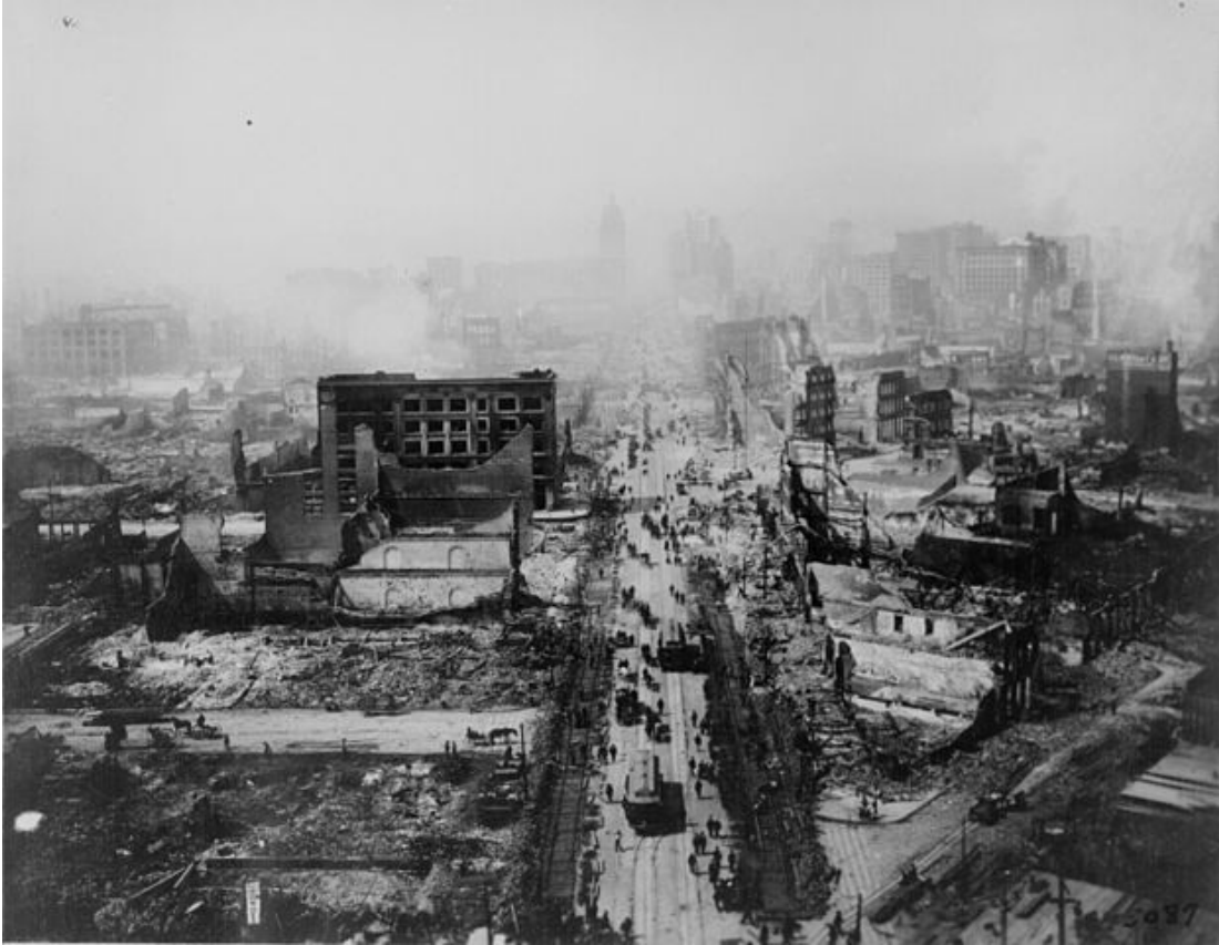
San Francisco Earthquake 1906
