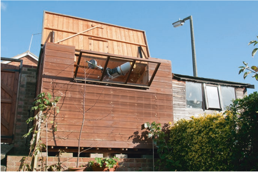
Fig. 2.3 Positioning your observatory – a battle of lights, horizons and garden plants! This observatory is sited at the top of a sloping garden and accessed by a series of steps. The side panel drops down to provide a good southern horizon, and the roof partly blocks a very annoying and inconsiderate street lamp! (Image by Andy Gannon)
