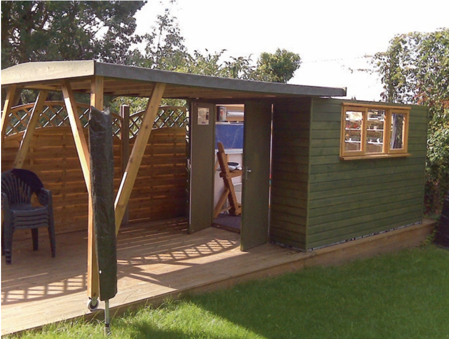
Fig 2.5 A roll-off roof 3 m by 2.5 m (10 ft by 8 ft) observatory is sited in the north-west corner of the owner's garden. This affords better views to the darker northeast section of the sky and is only partly impacted by the wire fence. The tree to the west has since been removed, revealing more of the light dome from London positioned south and west. (Image by Malcolm Zack)
