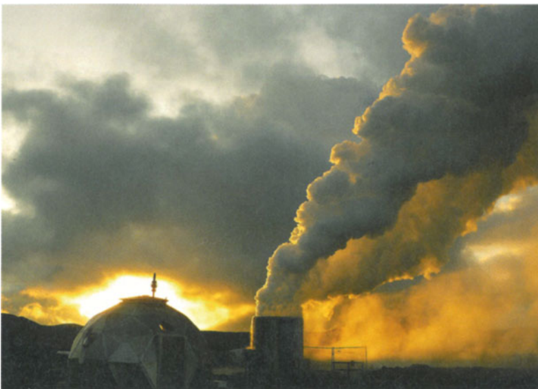
1.7 Hot water from inside the earth as an energy source: Well HE-53 in the Hellisheiði geothermal field in South-West Iceland during a production test.
