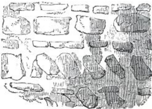
Rubble Masonry, from Gundulph's Tower, called St. Leonard's, at Malling, Kent, A.D. 1070.
