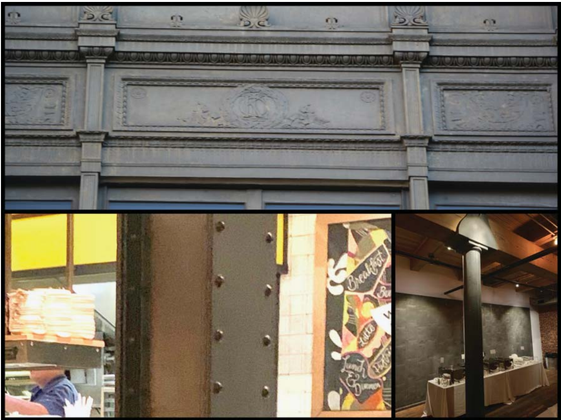
FIGURE 1.7 Cast iron columns and curtainwall.
