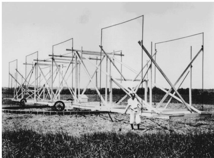
**Fig. 1.2** The “merry-go-round” antenna. Its creator, Karl Jansky can be seen right of centre. (Image courtesy of NRAO/AUI)
